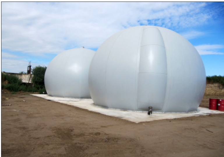
Gazometre biogaz
